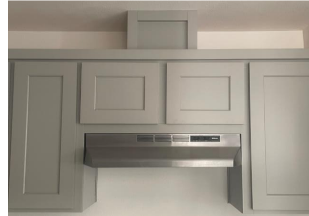
Cabinet Crown Molding
