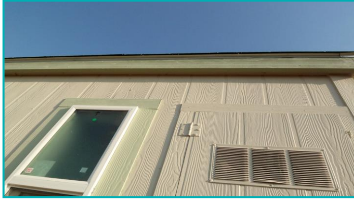
Rough Sawn Fascia
